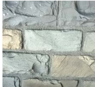
Grout based on VARIODUR 50 at the Höllenbach viaduct
