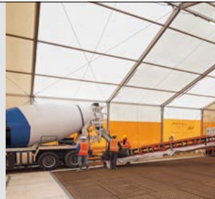
Application of high-strength concrete ...
